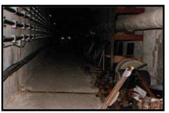
The tunnel viewed from the far end. Purely for information, on the left side of the figure, we can see the old water pipes supplying the University and on the right side the 3 phase power cabling. The useable tunnel length for our measurements is about 70 metres (one way), and we are about 5 metres below ground. The average temperature, during both summer and winter, is about 15°C and the humidity is very high.
